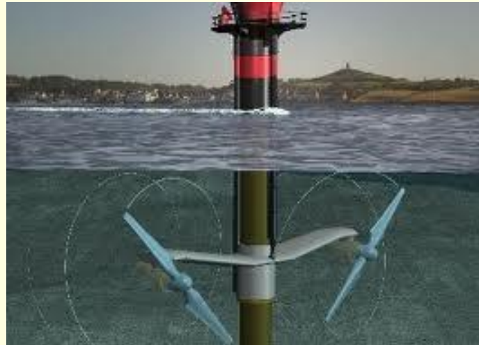
Ocean current power station in Northern Ireland (1.2 MW)
